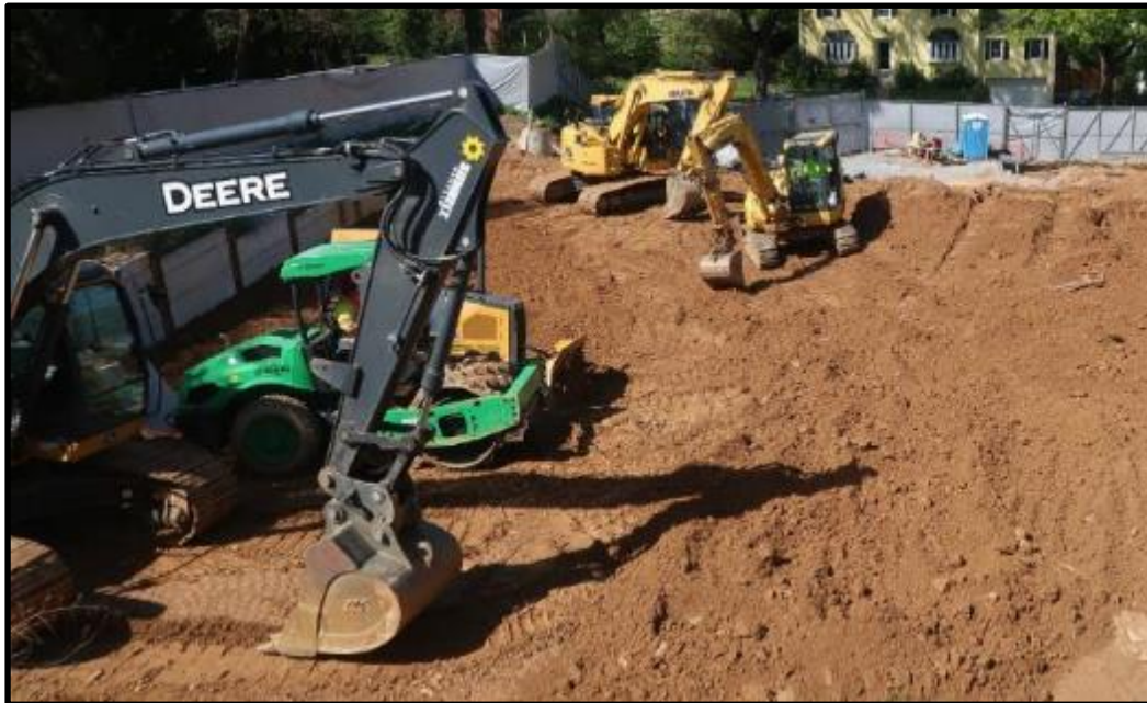
Spreading backfill around the site to dry.
