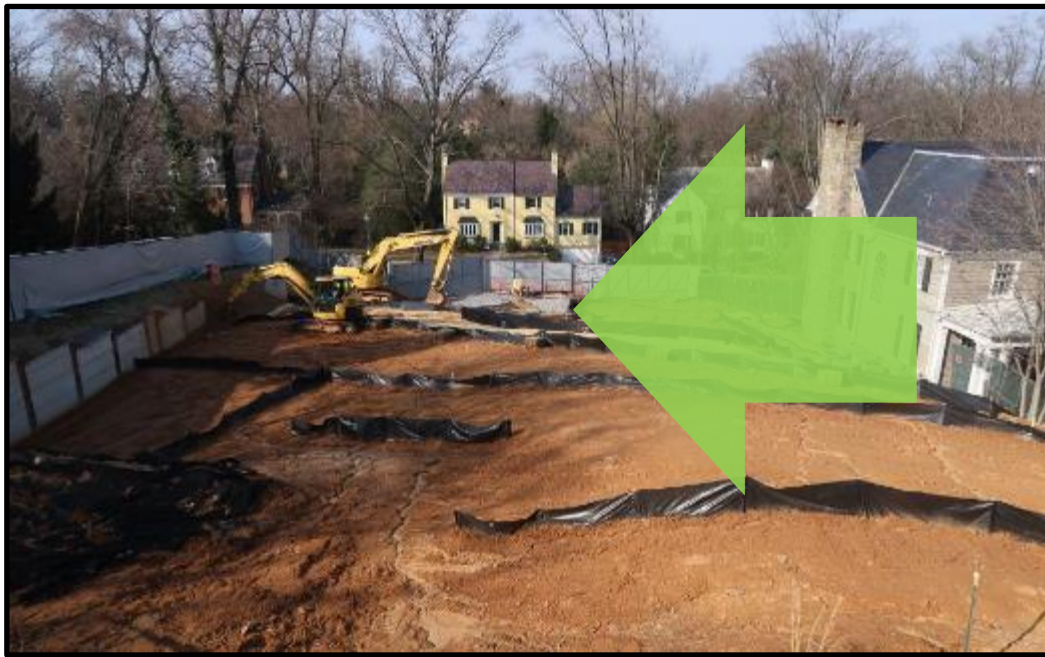
Site backfill progress from mid- March to first week of May.
