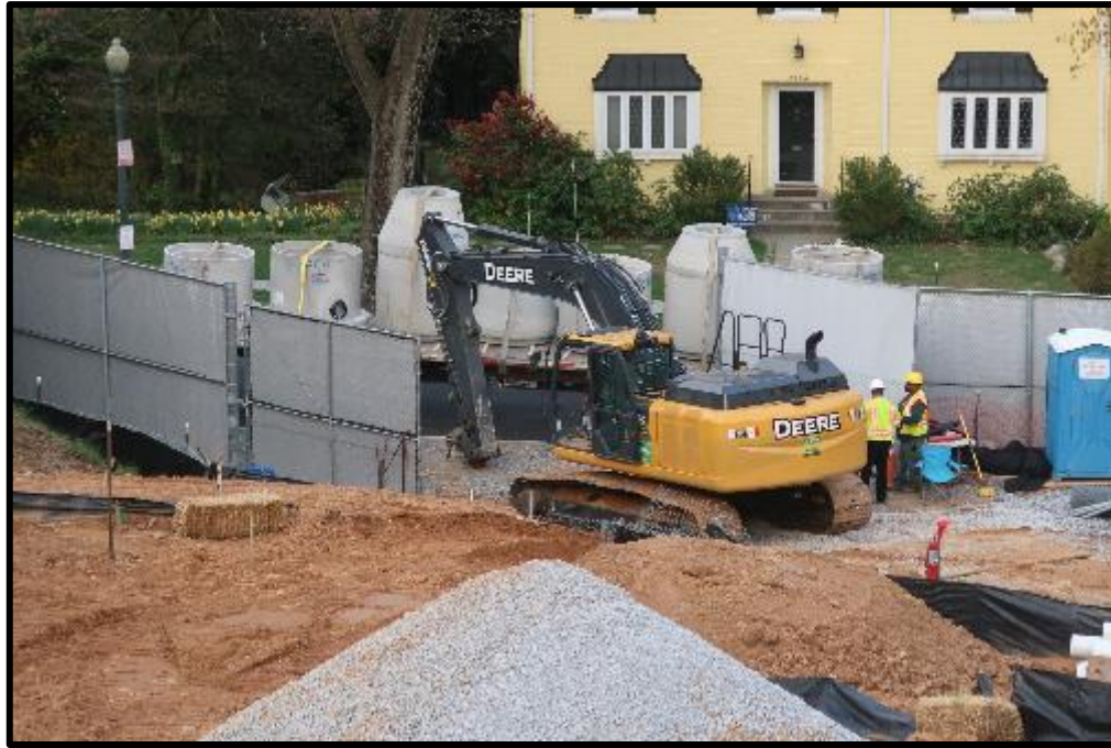
Materials being unloaded in April for the utility reinstallation effort.
