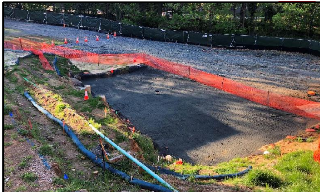
Restored Former PSB excavation site
